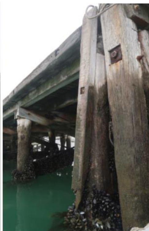
Failed vertical fender to pile 28A, timber fender is twisted about single remaining fixing
