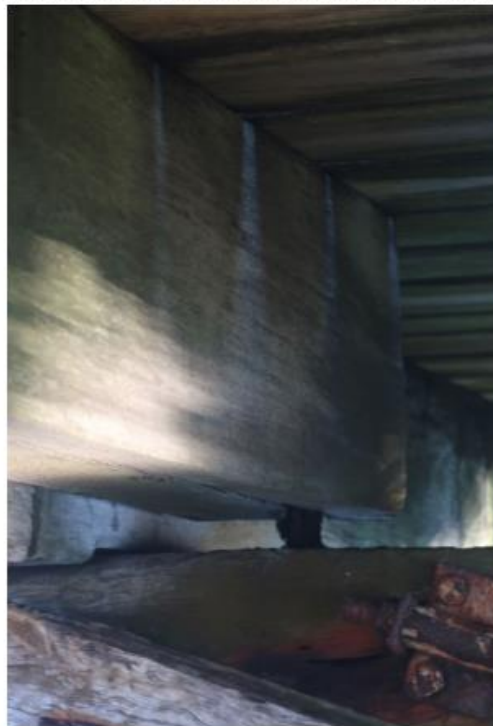
Poor seating to stringer g on bent 26-27. Both ends require packing to fill gap to cap beam
