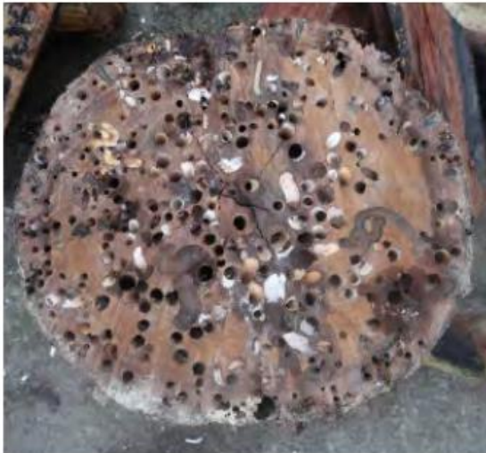
Figure 11: Marine borer damage to hardwood pile
