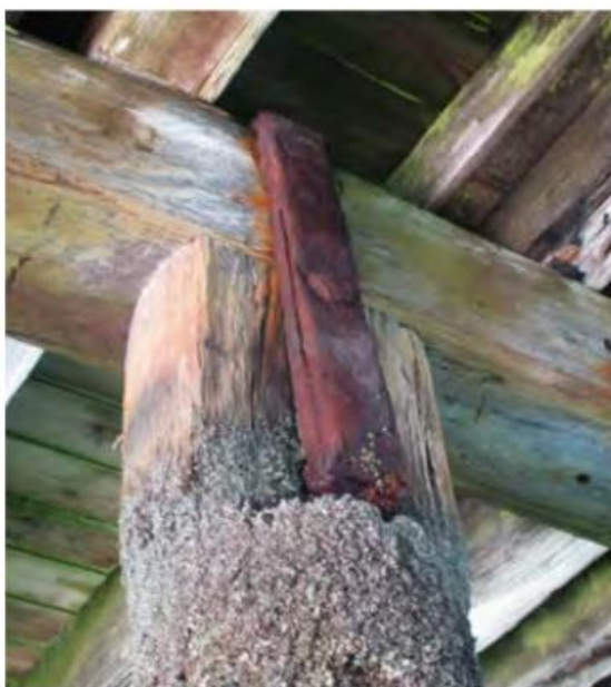
Figure 6: Corrosion to fixing at top of pile. Fixing consistent with original 1878 detailing.
