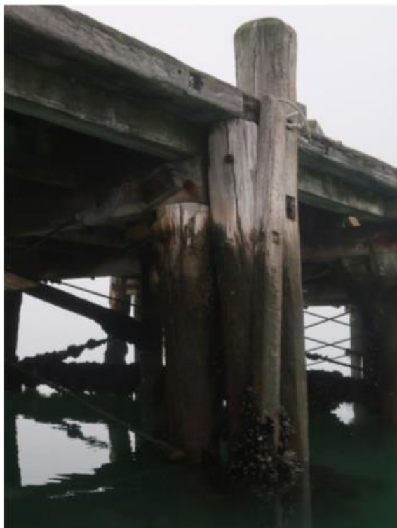
Failed vertical fender to pile 28A, timber fender is twisted about single remaining fixing
