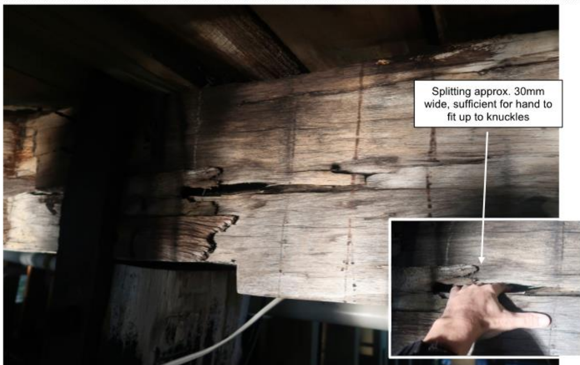
Severe splitting to cap beam over pile 14D, below Black Cat building
