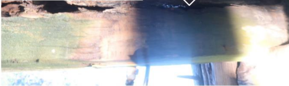
Severe splitting to outer stringer g, bent 27-28. Split approx. 1.5m long through width of section
