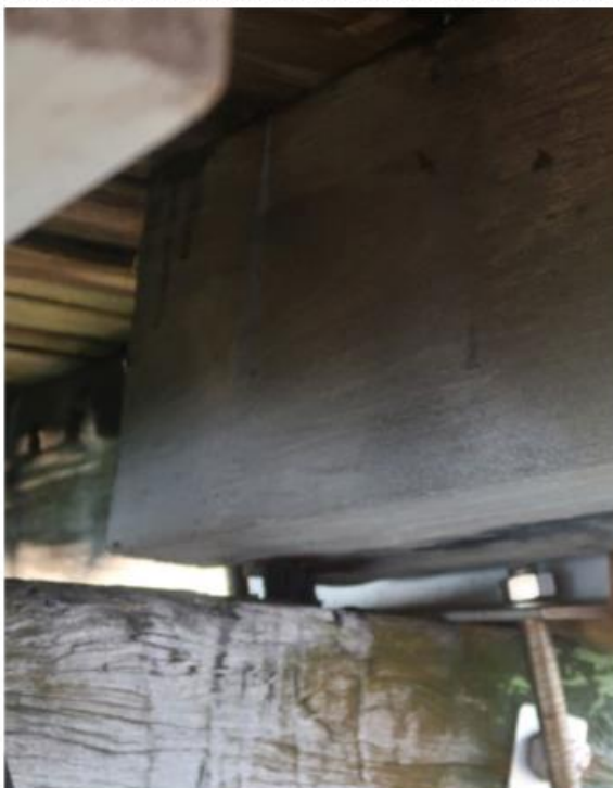
Poor seating to stringer g on bent 26-27. Both ends require packing to fill gap to cap beam
