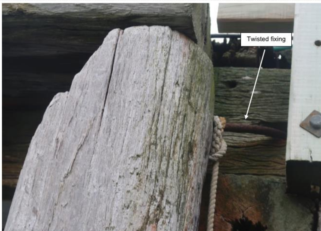
Poor connection at top of fender pile at grid 27C. Severely bent bolt fixing visible to the right of pile.
