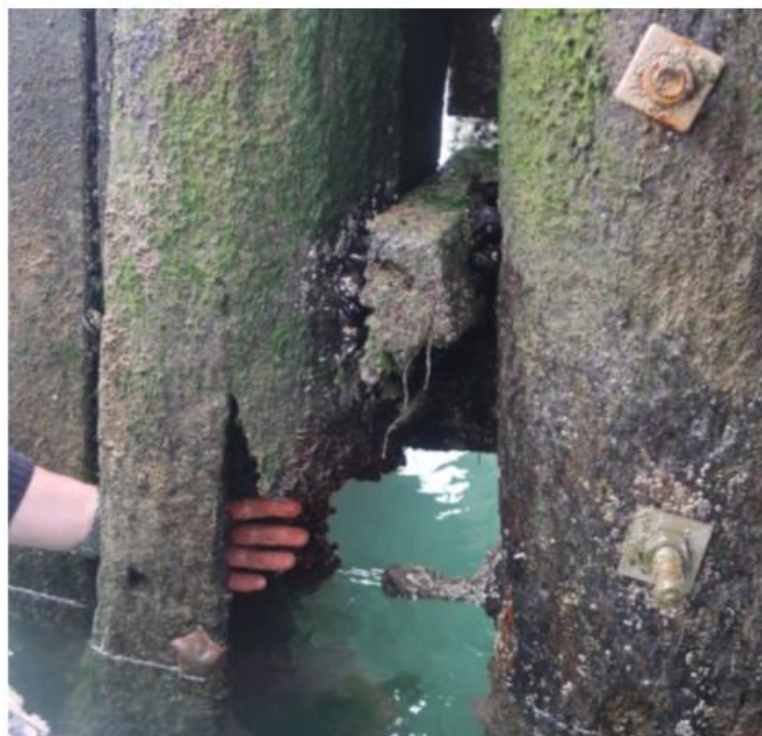
Failure of fender pile 26A at low water line
