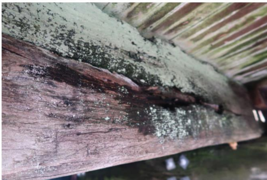
Severe rot and splitting to stringer b, between bents 11 & 12
