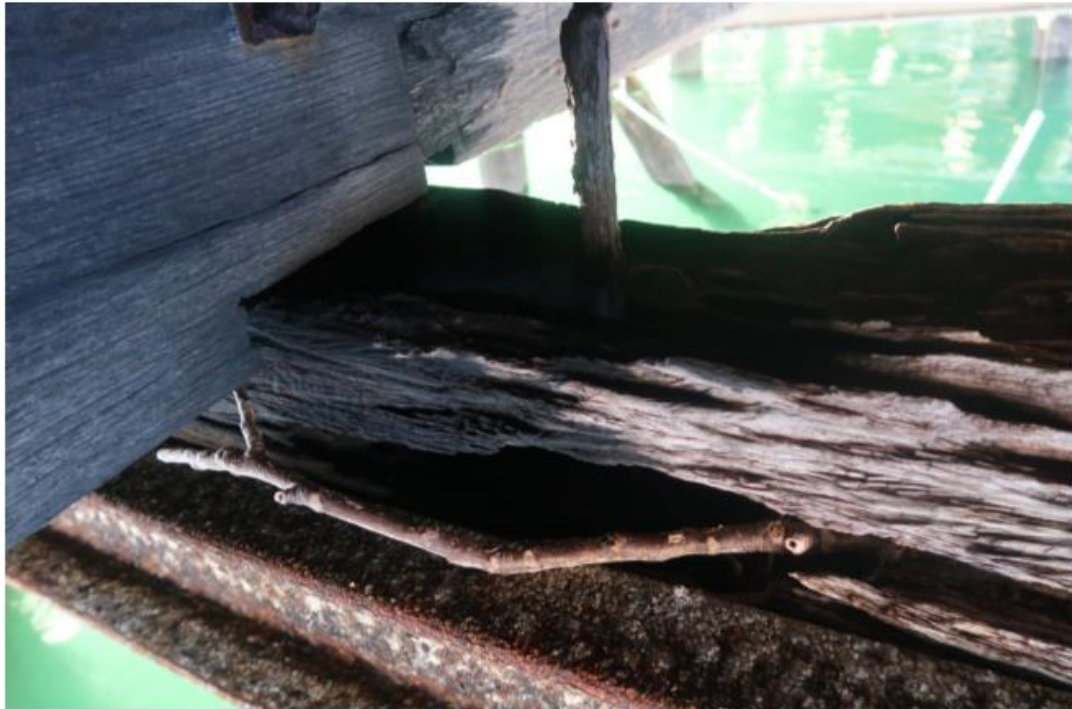
The timber cap beam is in extremely poor condition, there is more recent steel PFC beam which has moderate corrosion, but this is not supporting the stringer beam above. Area near pile 20C below Blue Pearl building
