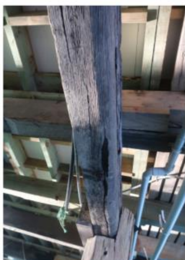
Severe splitting to cap beam along gird line D, between bents 11 & 12, below Black Cat building
