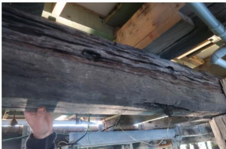
Severe splitting to cap beam along gird line D, between bents 11 & 12, below Black Cat building
