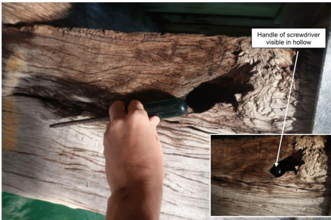
Cap beam on grid 19, severe hollowing. There is a large void, which the entire screwdriver could fit in
