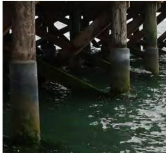
Figure 12: Timber piles with FRP jackets
