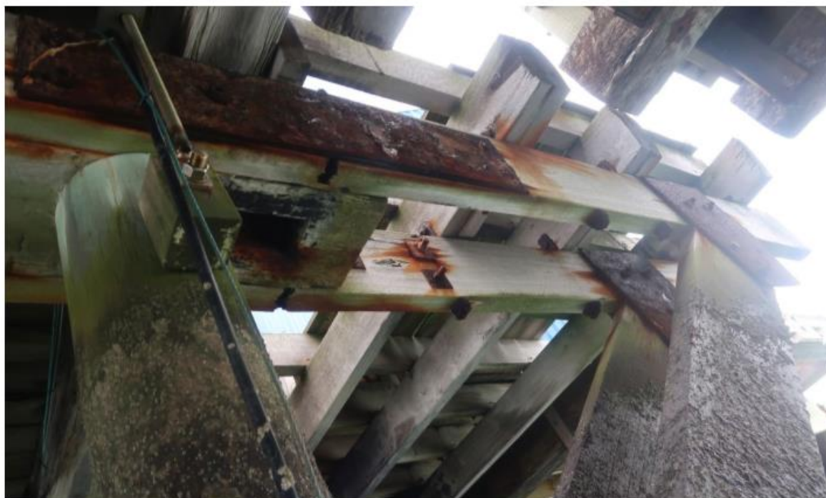
Cap beam at pile 21C, supporting northern end of Blue Pearl Building. Old splice repair in poor condition
