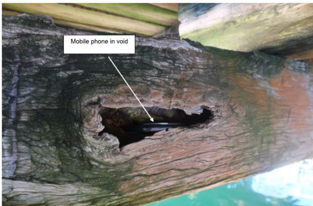
Cap beam on grid 26, large hole in beam.
