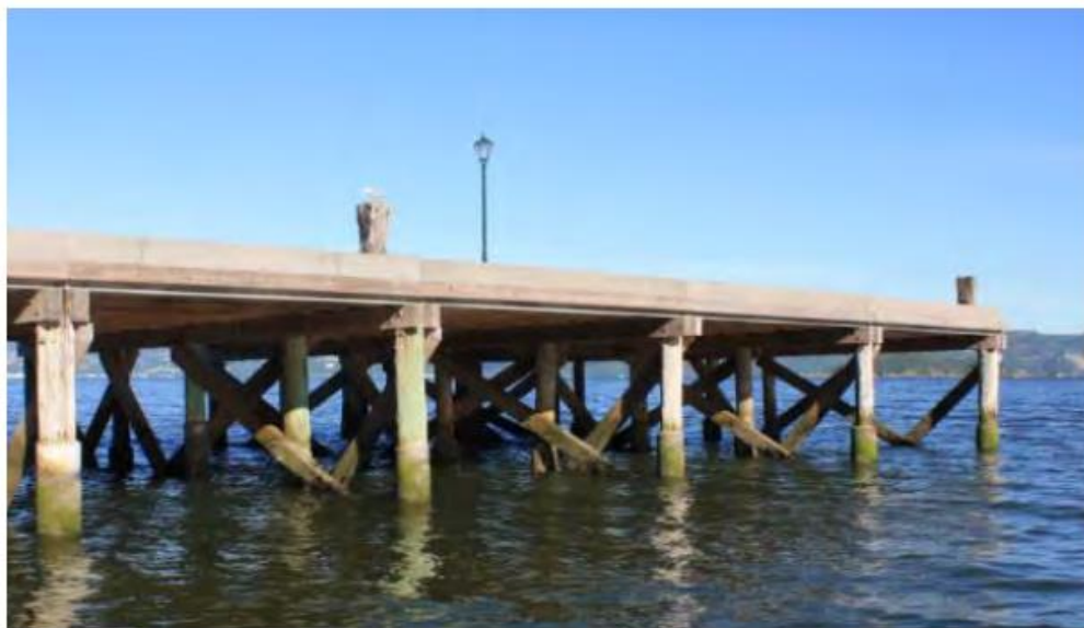
Figure 20: Rona Bay Wharf, timber piles and bracing with concrete edge beam and deck
