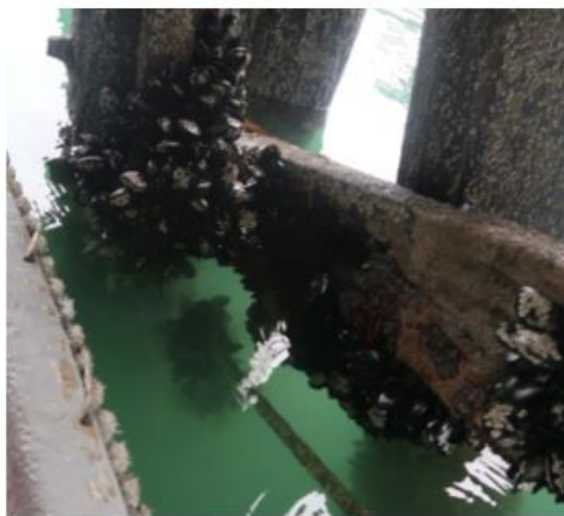
Failed Bracing to bents 21 (left) & 22 (right)
