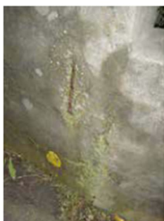
Damage caused by rusting reinforcing.
