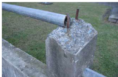
Spalling plasterwork and missing top section of post
