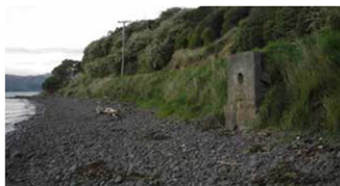
Concrete foundation for culvert (Mosley, May 2010)
