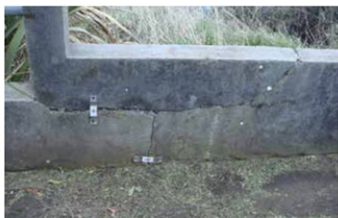
Cracks in concrete surrounding wall. Note "telltales"
