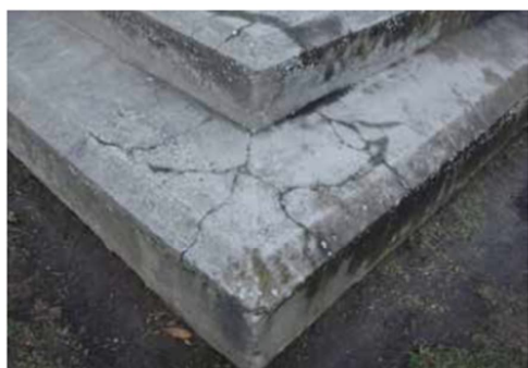
Base of monument showing cracking
