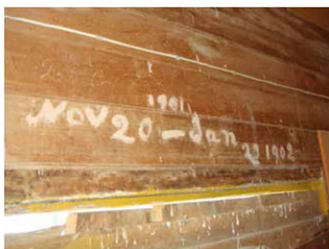
Barracks interior. Note tongue and groove wall linings and metal tie rod spanning the width of the building
