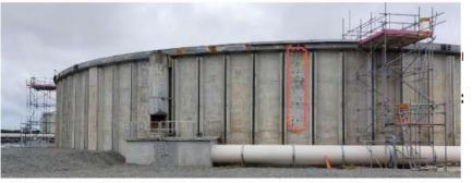
Trickling Filter 2 showing scaffold towers constructed for access to carry out assessments and concrete samples taken (outlined in red)
