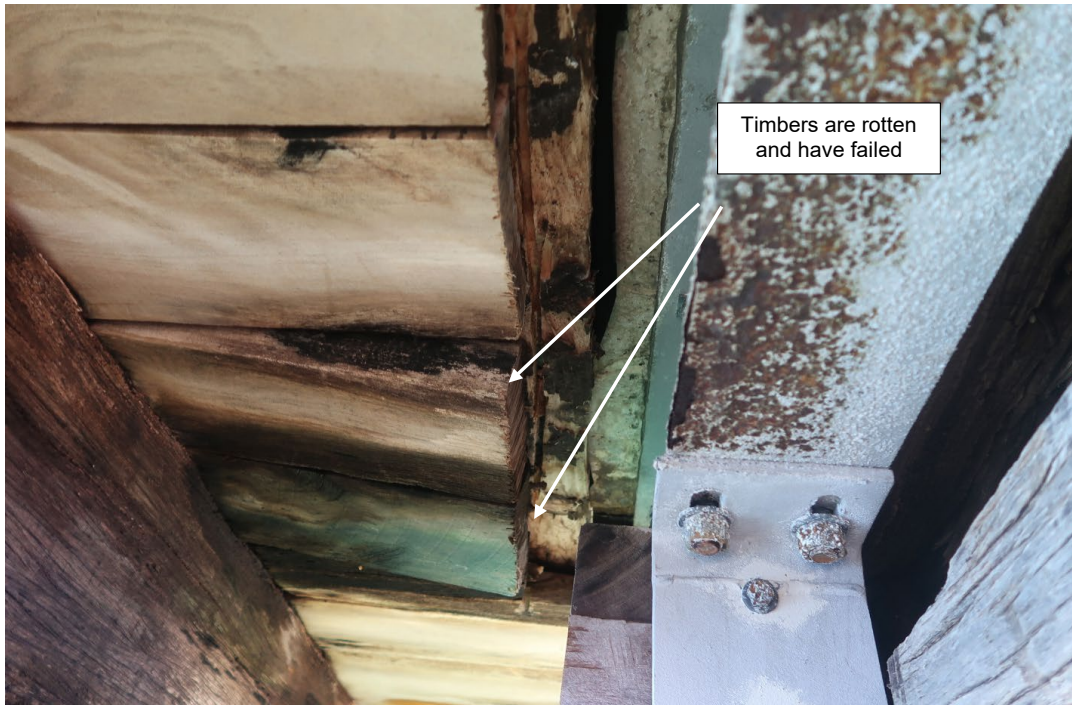
Rot to timber below concrete deck between bents 17-18. Two deck timbers have failed and have dropped away from deck.
