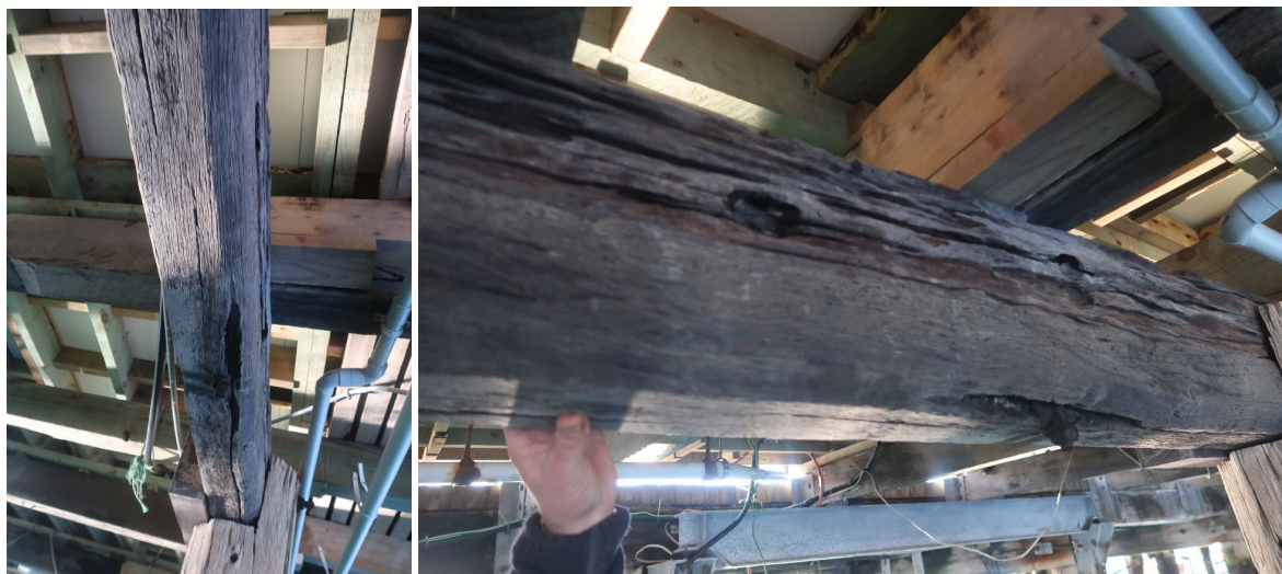
Severe splitting to cap beam along gird line D, between bents 11 & 12, below Black Cat building
