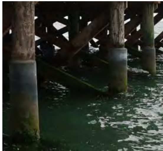
Figure 12: Timber piles with FRP jackets
