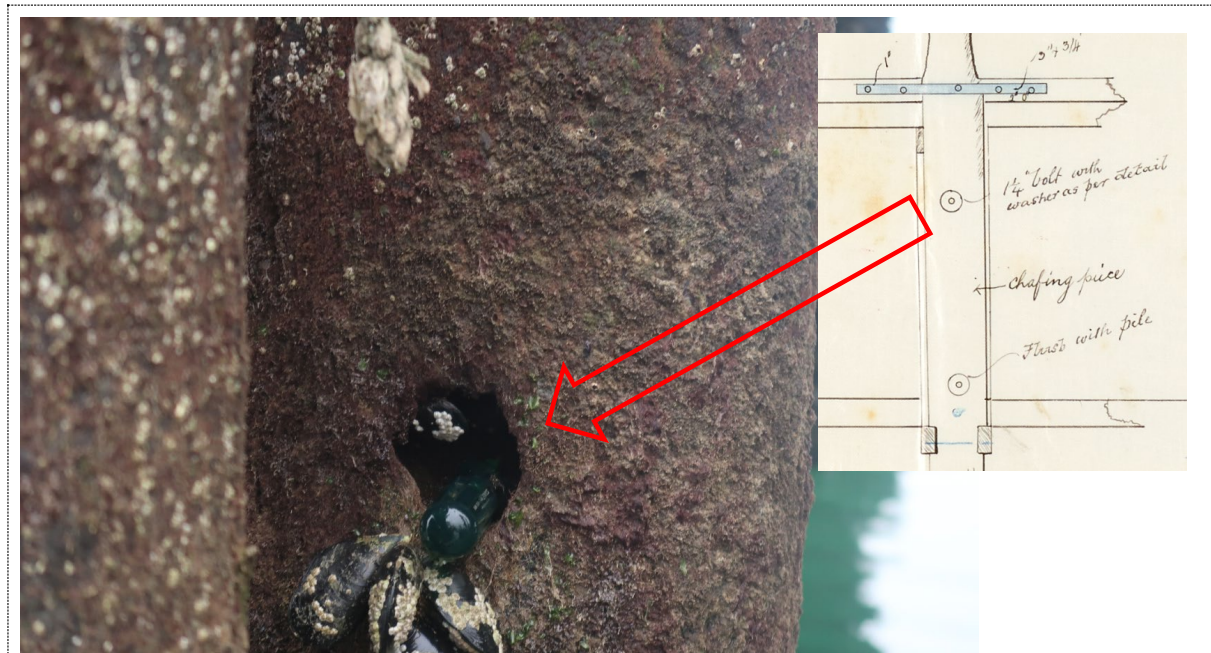
Typical hole approx. 70mm Ø in intertidal zone on an original vertical pile, extract from original construction drawings showing hole is consistent with where fixing was located.
