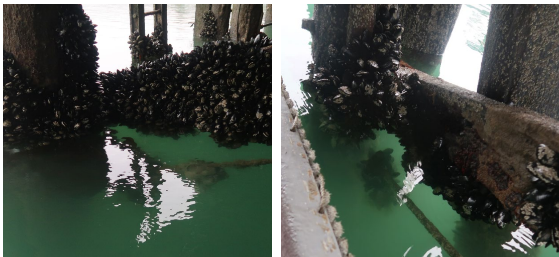
Failed Bracing to bents 21 (left) & 22 (right)
