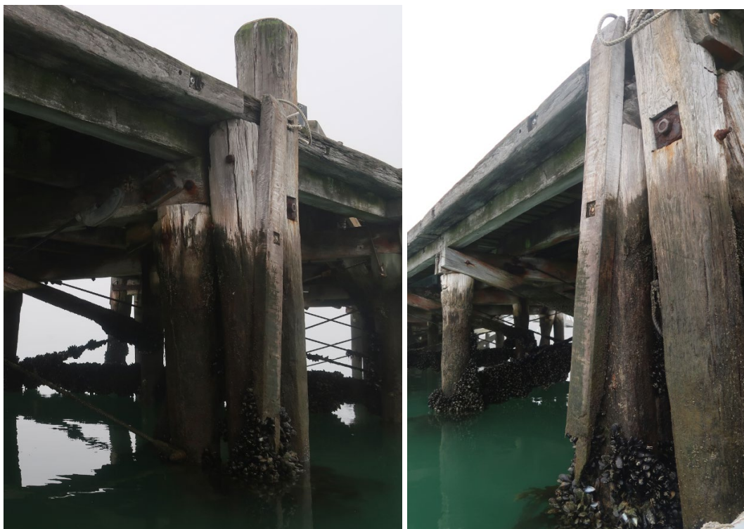
Failed vertical fender to pile 28A, timber fender is twisted about single remaining fixing
