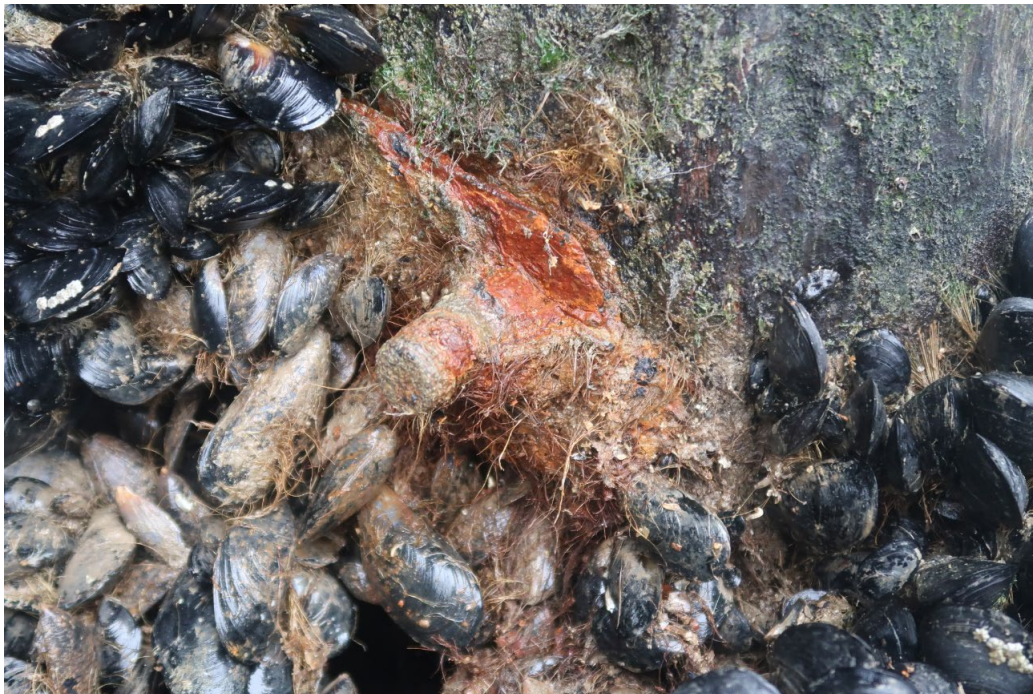
Lower bracing connection to pile 27A, bracing close to failure due to severe corrosion
