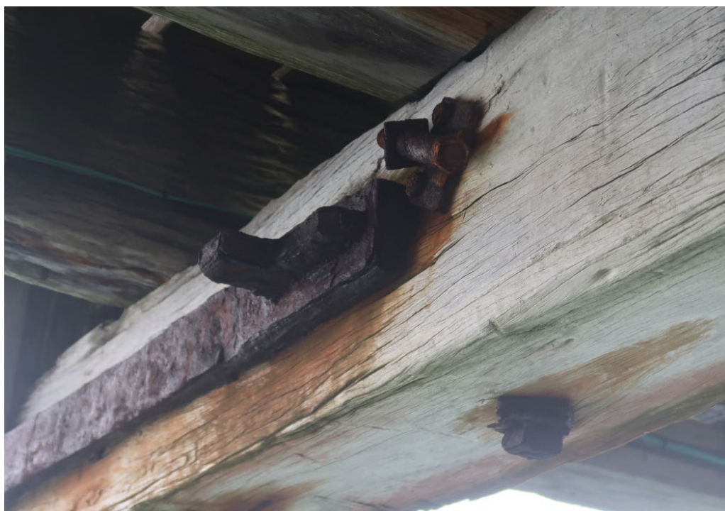
Top of pile 24A Failed tension bracing. Note, original iron connection detailing present to pile cap and fender pile
