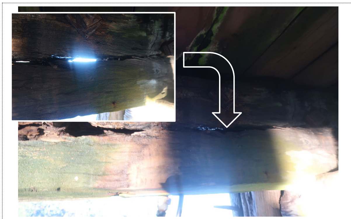
Severe splitting to outer stringer g, bent 27-28. Split approx. 1.5m long through width of section
