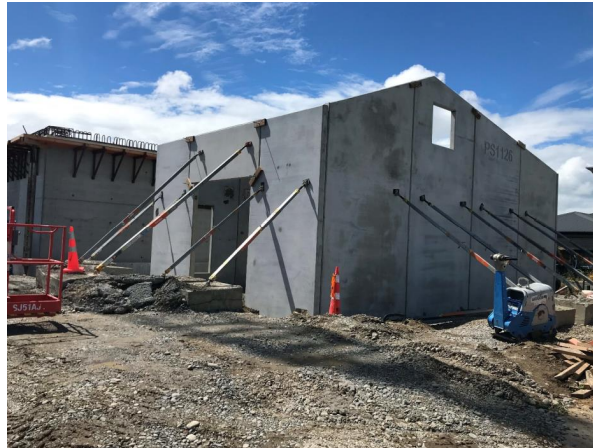
Pump station building (foreground) and suction tank (background) at Ben Rarere PS.
