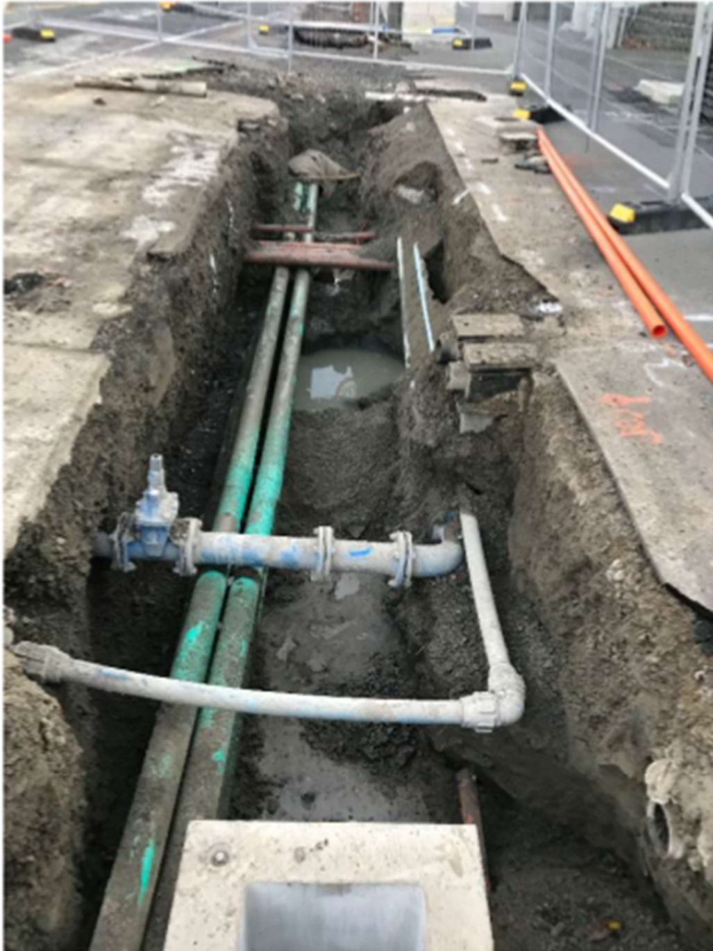
Working around existing services, very complex and slow
