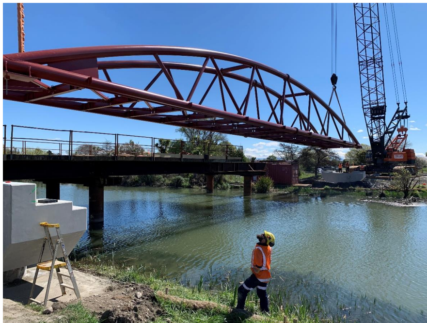
Avondale Bridge being emplaced
