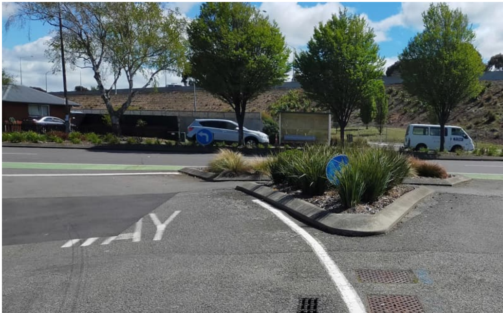
Figure 14: Nairn Street (keep left sign obscured, no give-way sign in island, no KTMs)
