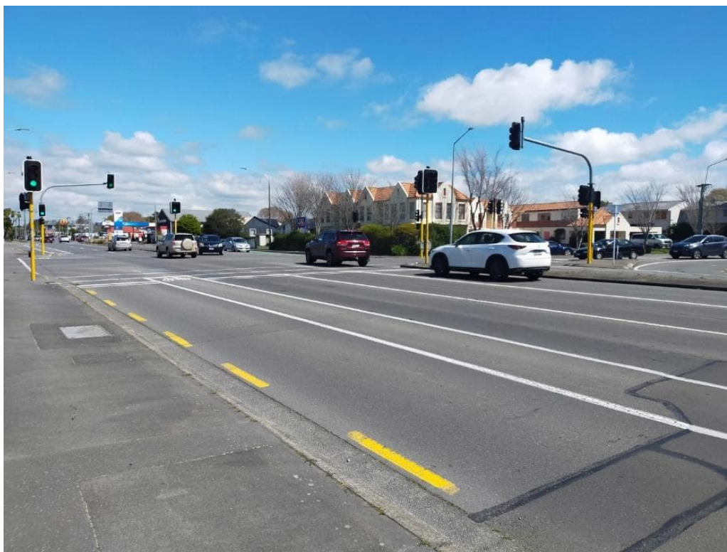
Figure 39: Lack of green surfacing in cycle lanes at major intersections
