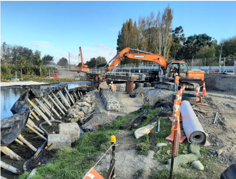
Gabion Wall construction North side of River
