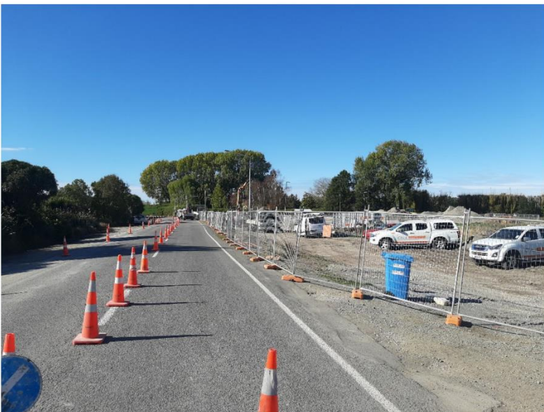
Lower Styx Rd, Service trench installed, overhead power lines removed, new light poles installed
