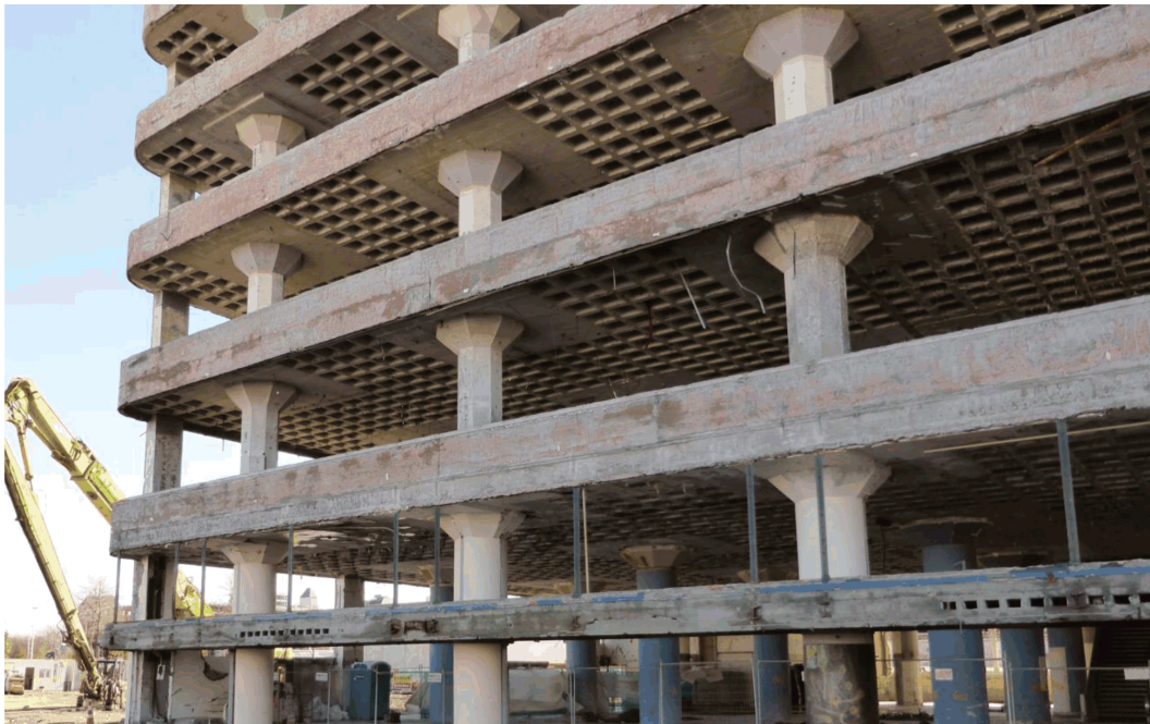
Demolition of former Millers Building 2014: massive innovative concrete construction 1939
