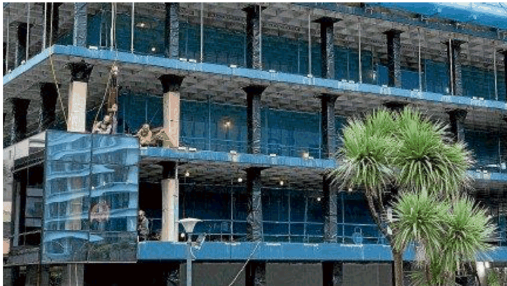
Window units being installed during the redevelopment of Wellington's Charles Fergusson tower.
