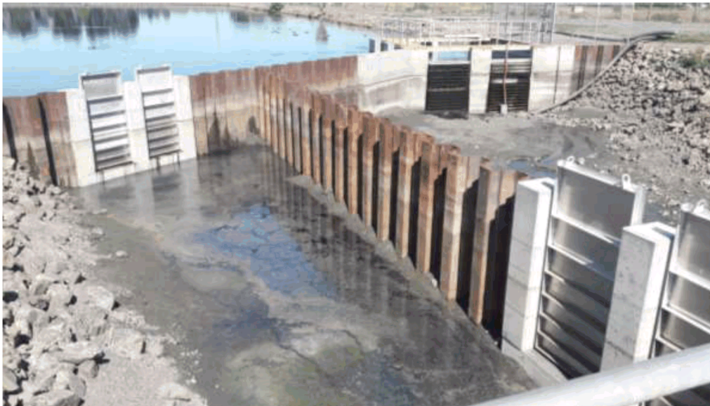
Photograph showing the new civil structures installed (center & top left) which allows the flow through Oxidation Ponds 1 & 2 to be reversed (previously an open channel)
