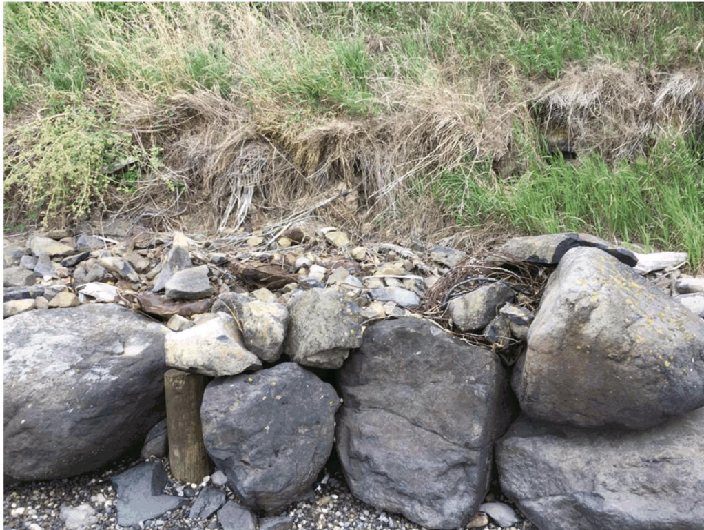
Figure 4. Small section of seawall at Barry's Bay closed landfill requiring repair.
