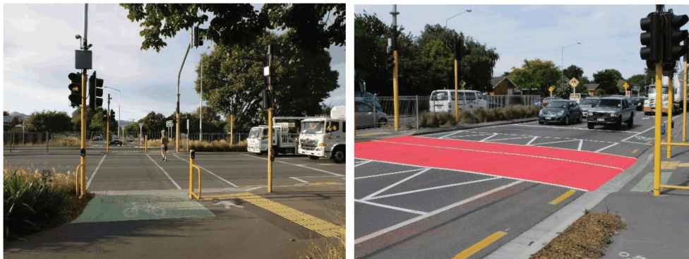
Figure 1: (Approximately) compliant vehicles before and after the changes to the crossing. As well as the colour marking, the stop line is 1.5 m further back from the crossing.
