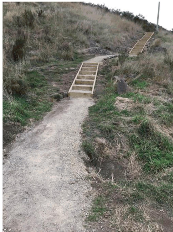
Two flights of wooden stairs and material including shingle brought in to form urbanised path
