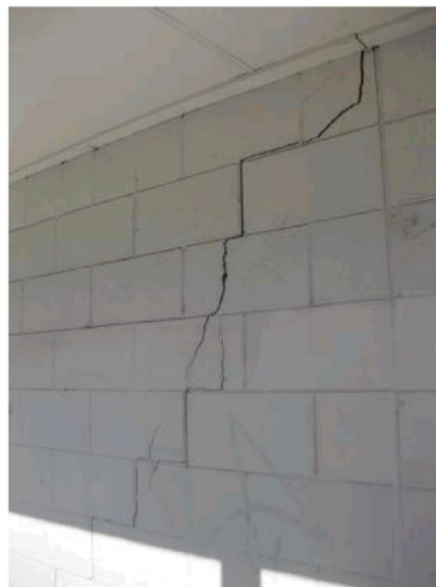
Photo 6: Crack in the front wall
