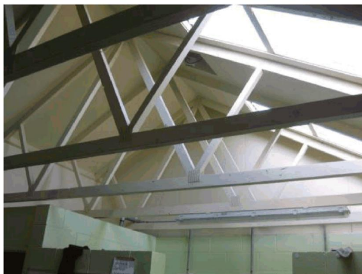
Photo 9: Roof truss and lining
