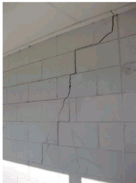
Photo 6: Crack in the front wall
