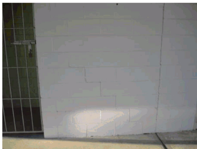
Photo 8: Diagonal crack in the front wall
