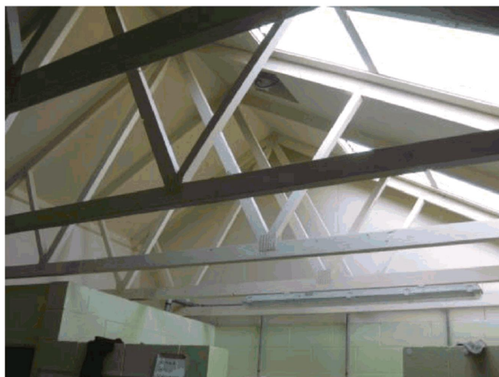
Photo 9: Roof truss and lining
