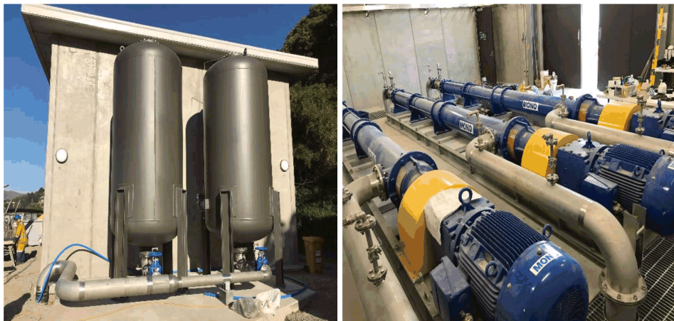
Left, pressure vessels at Simeon Quay PS, right: progressive cavity pumps at Power House behind Simeon Quay PS
