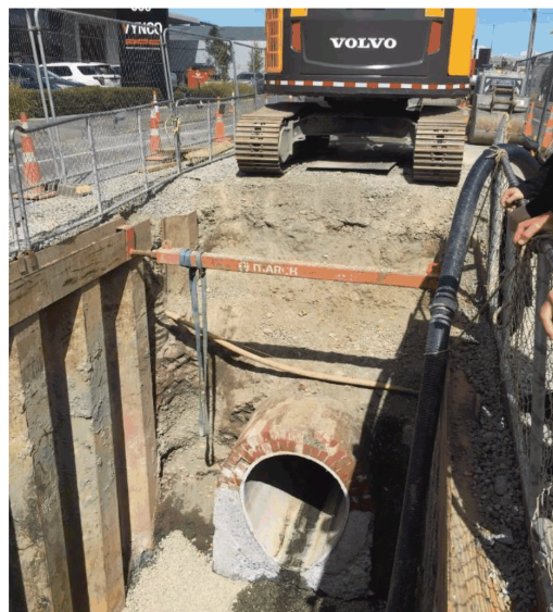
Tuam Street Brickbarrel – Portion of existing pipe to which we are connecting.
