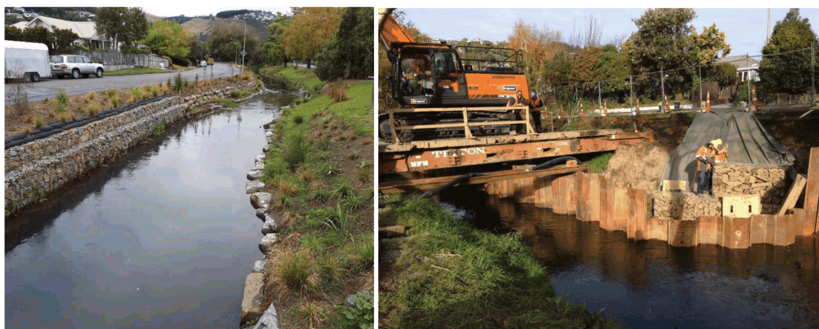
Figure 2. Palatine/Eastern Terrace (left) and gabion wall construction at 36 Centaurus Road (right)
