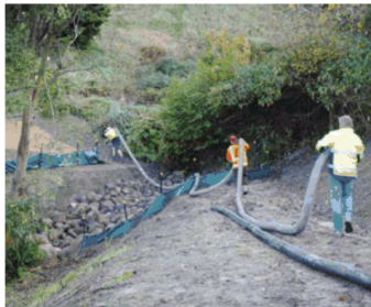
Blanket applied pneumatically over loess clay base
