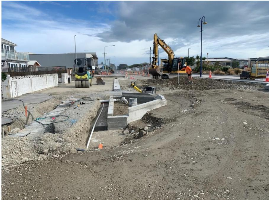
*New V Channel, kerbing and one of the rain gardens on Eastern Side, preparation for Road carriageway*
