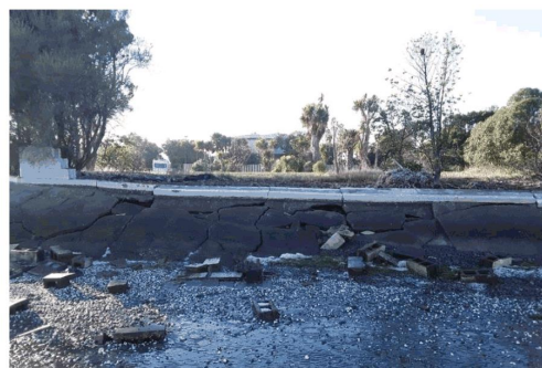
Figure 28: Structure IS32 – 9 Kingfisher Lane (Area 5b) a) in 2002 showing a “satisfactory” seawall (ECan, 2002), and b) in 2019 with structure condition grading ‘D’ (Jacobs, 2019 image).
