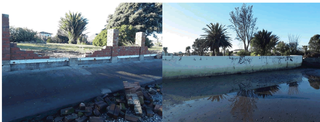
Figure 30: Examples of structure condition grading 'D': a) Structure ISIS1 – 126A Rockinghorse Rd (Area 5c); b) Structure ISIS14 -136B Rockinghorse Rd (Area 5d). (Jacobs 2019 images)
