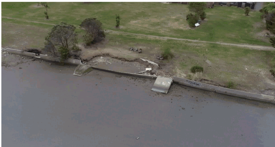
Figure 37: Structure IS23-A, Variable remnant structure elevations- Wall sections above 11.2m, and low foundation sections 10.25m with 3.5m of erosion behind.
