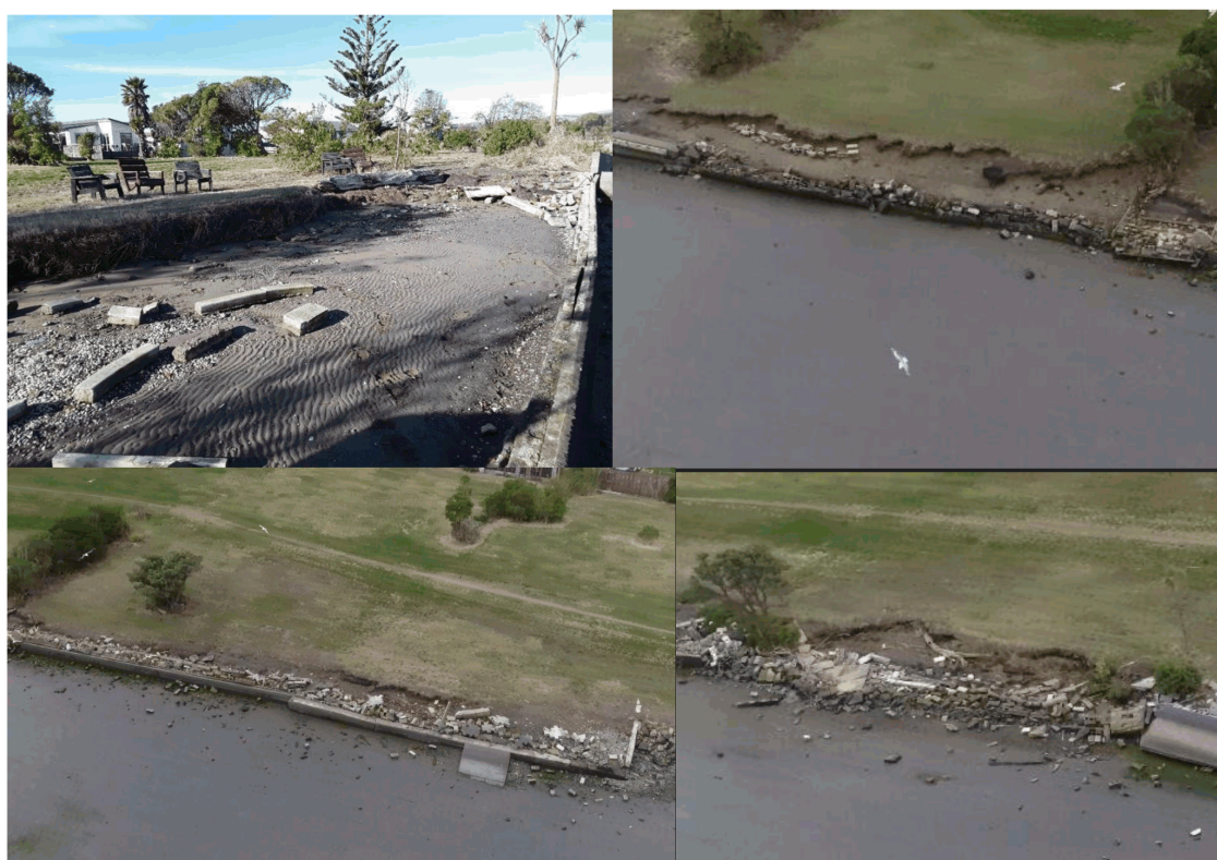
Figure 43: Location of significant erosion scarps behind remnant wall structures between Penguin and Plover Streets (Area 5c) a) IS23-A, erosion 3.5m; b) IS22-F, erosion 2.3m; c) IS22-E, erosion 2.7m; d) IS22-A, erosion 2.8m.
