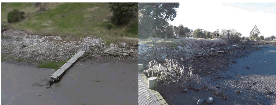
Figure 42: Location of informal fill between Heron and Penguin Streets (Area 5b) with 2011-2019 erosion >4m. (image a) from ECan Drone, 2019; image b) Jacobs, 2019).
