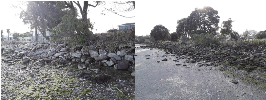
Figure 41: Locations of informal fill between Godwit and Heron streets (Area 5a) with 2011-2019 erosion >4m a) Structure IS39-A, immediately south of Godwit St, and b) Structure IS23-A approximately 90m south of Godwit St. (images Jacobs, 2019).
