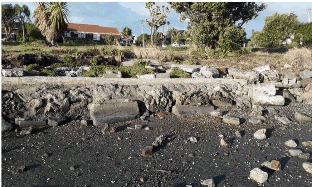
Figure 5: Structure IS10 - low lying concrete wall, condition graded 'D' rather than 'E' due to still providing some functionality against erosion (Jacobs, 2019)
