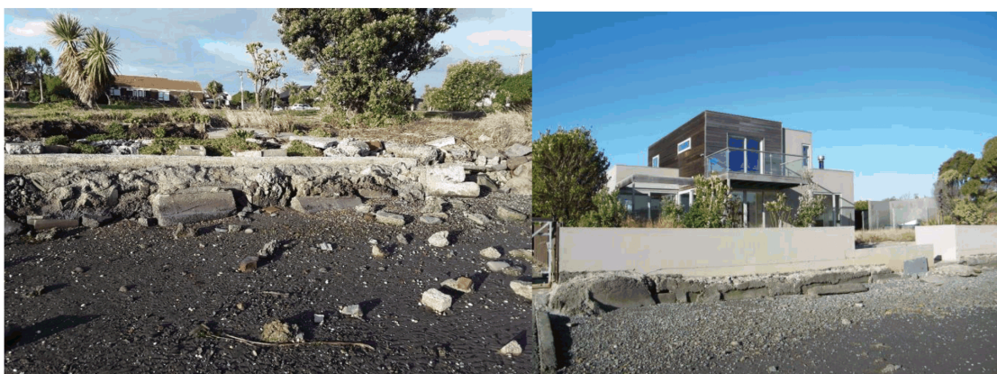
Figure 38: Structure IS10-A: a) 2019 low elevation foundation remains of former concrete wall (Jacobs 2019); b) Current structure elevation 10.6m, structure condition 'D', land condition 'D' ( A. Crossland 2014).
