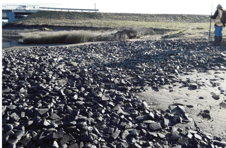
Figure 12: Informal rock revetment (IS47-A) south of South Bridge Street
