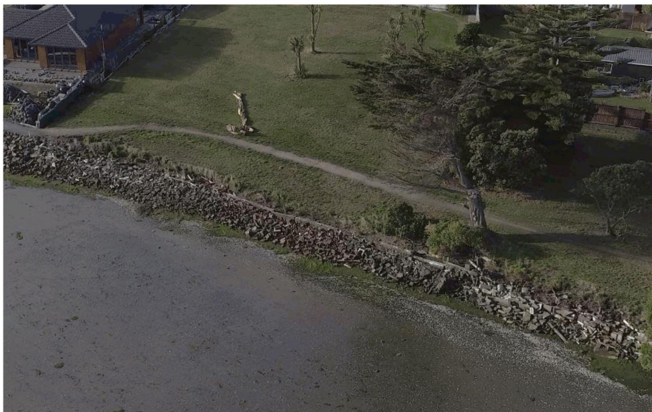
Figure 33: Structure IS34-A north of Heron Street, lowest structure elevation of 10.46m and average of 10.82m. Structure condition grading 'C' and land condition grading of 'D'
