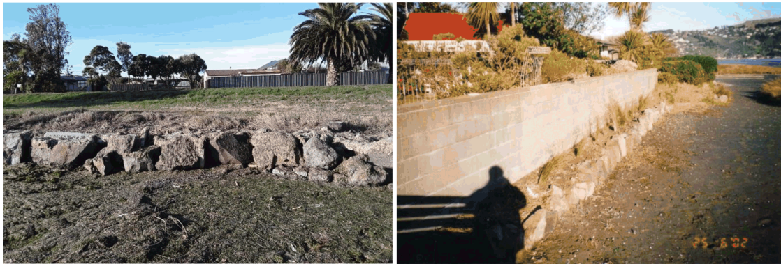
Figure 35: Structure IS26. Minimum 2019 structure elevation in Area 5b. a) 2019 condition -single line rock revetment; b) 2002 concrete block wall above rock revetment. Current land condition 'D'.
