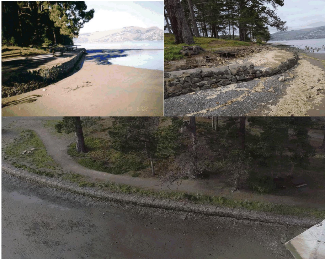
Figure 16: a) Masonry wall south of jetty in South New Brighton Park in excellent condition in 2002 (ECan 2002); b) wall failed and erosion behind in 2017 (Jacobs Image); c) replacement gabion wall (GB3-A & GBRM3-A) in June 2019 (ECan drone image)
