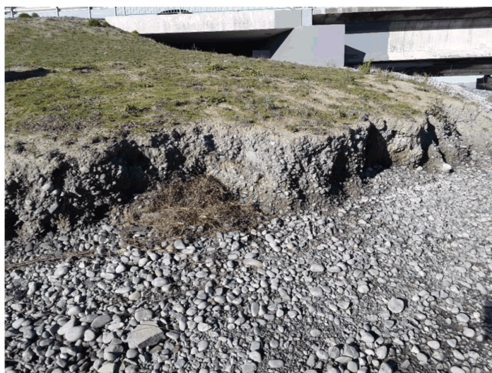
Figure 9: NS17-A Land condition 'E' – 0.6m erosion scarp on grass embankment north side of Bridge St.
