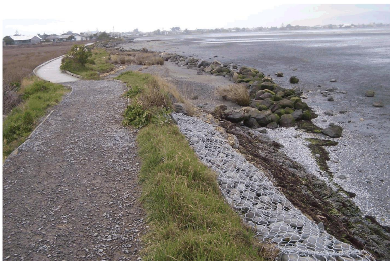
Figure 17: Reno mattress (RMRV1, RM1-A) in good condition at north end of Jellicoe Marsh Boardwalk in 2009 prior to the CES (Image Supplied by A Crosslands, 2009)
