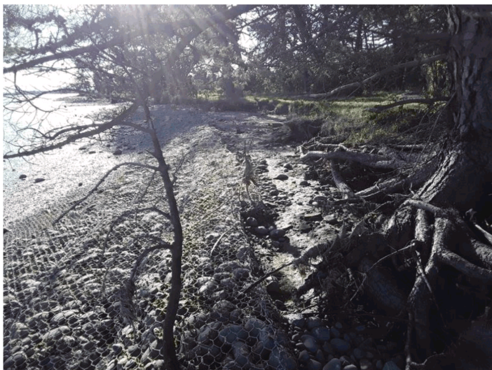
Figure 19: RM2-G Example of condition 'C' reno mattress with a condition 'E' coastline (Jacobs, 2019).
