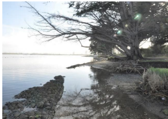
Example of reno mattresses that have slumped
