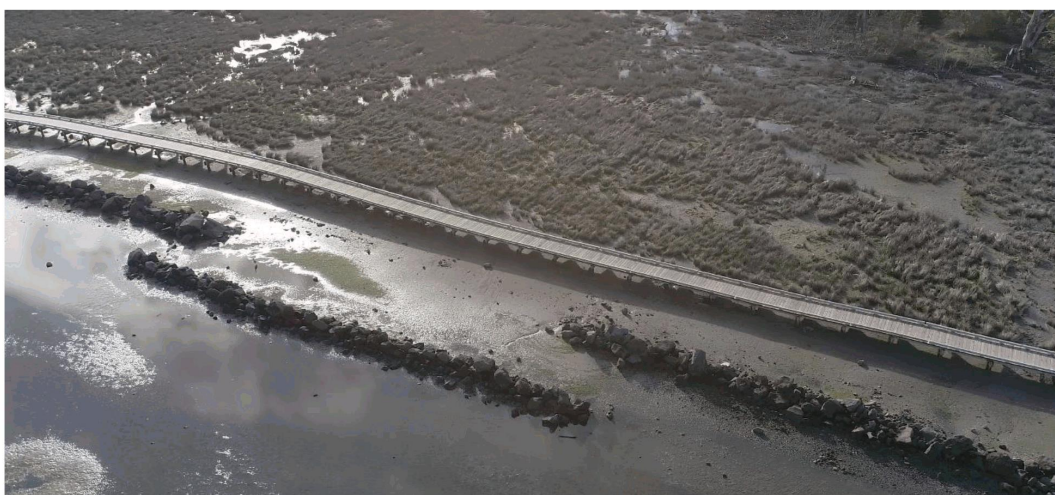
Figure 6: IS45-IS43 low lying revetment graded B* which have been put in place to break up wave energy to protect the boardwalk and salt marsh (ECan, 2019).
