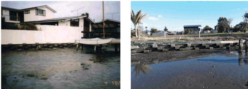
Figure 27: Structure IS7 -156B Rockinghorse Rd (Area 5e) a) in 2002 showing a seawall with 'Satisfactory' and b) in 2019 with structure condition grading 'E' (Jacobs, 2019 image).
