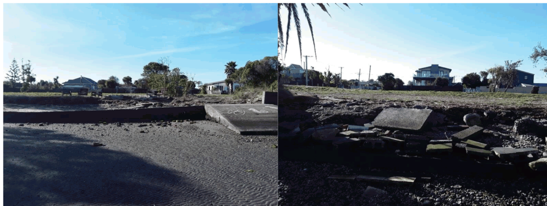
Figure 31: Examples of structure condition grading 'E': a) Structure IS23 – 104A Rockinghorse Rd (Area 5d); b) Structure IS20 – 4 Plover Street (Area 5d). (Jacobs 2019 images)
