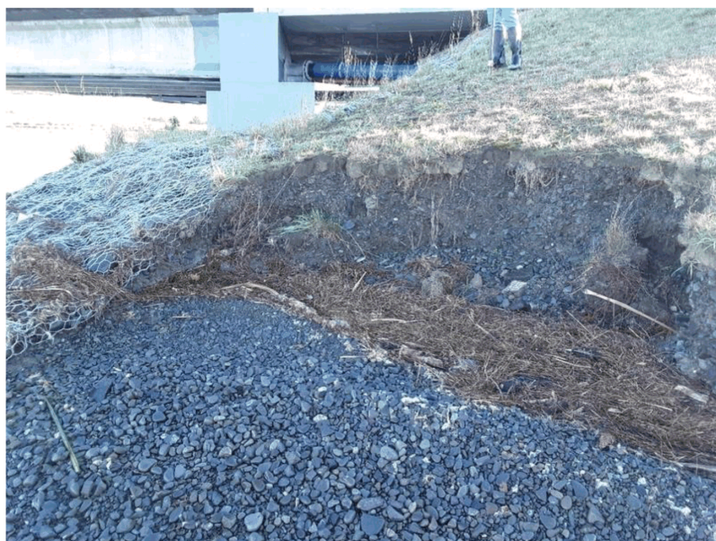
Figure 13: NS16-A Land condition 'E' – 0.6m erosion scarp on grass embankment south side of Bridge St.
