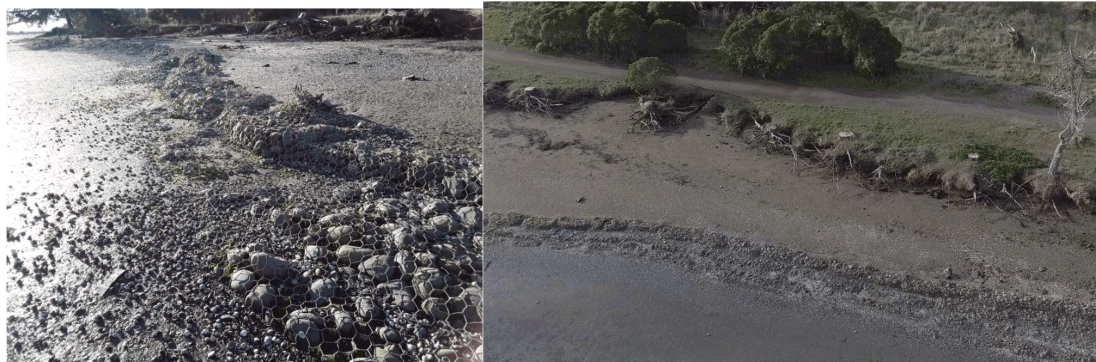
Figure 18: a) Condition 'E' reno mattress in Area 3 (RM2-I) (Jacobs, 2019 image); b) Land Condition behind the structure also graded 'E' due to significant erosion (ECan drone image, 2019).
