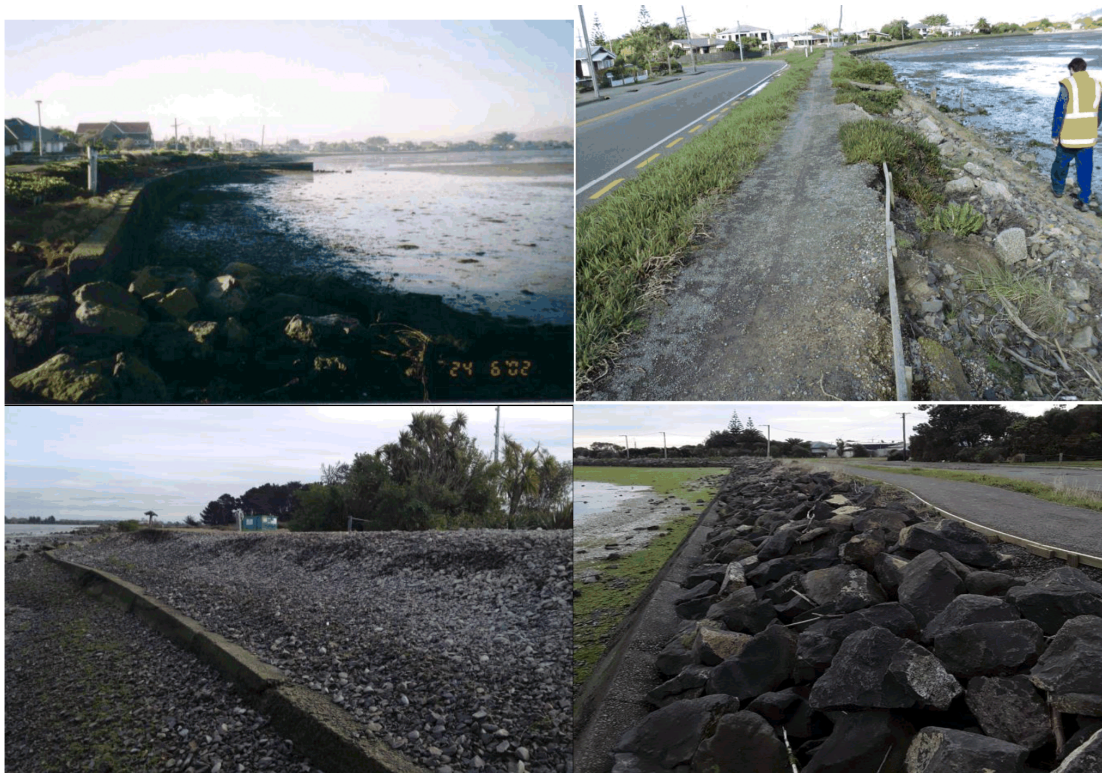
Figure 22: Ebbtide Street stopbank (SBW1-B): a) 2002 low concrete wall only (Ecan, 2002); b) Following the 4 th September 2010 earthquake (Christchurch City Council, 2010); c) Prior to placement of revetment July 2014 (Image supplied by CCRU) d) Current stopbank and revetment above original concrete wall (Jacobs, 2019)
