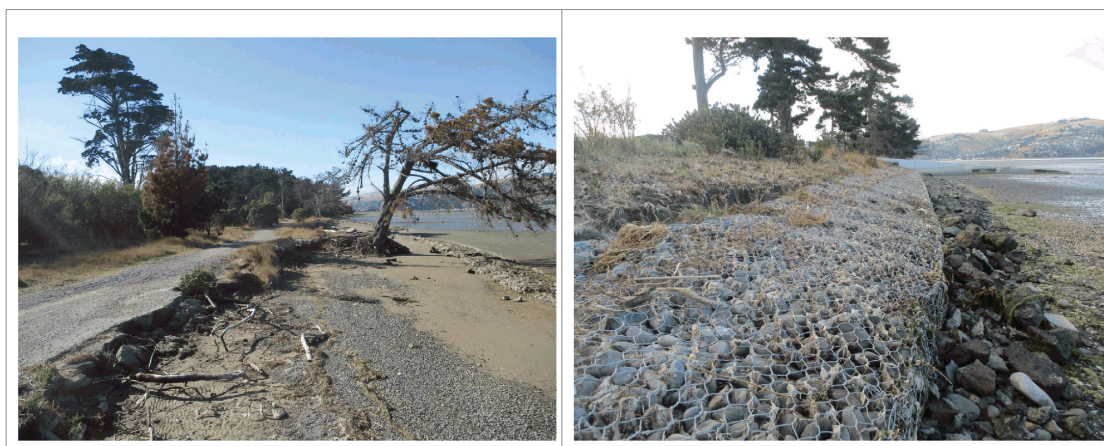
Figure 1.2: South New Brighton Park lies adjacent to the estuary, and is important to the community for its recreation, cultural, ecological, historic and business values. Reno mattress (cobbles within wire mesh) currently runs the majority of the shoreline of the Park from the South New Brighton Boat Ramp to the Jellicoe Marsh boardwalk
