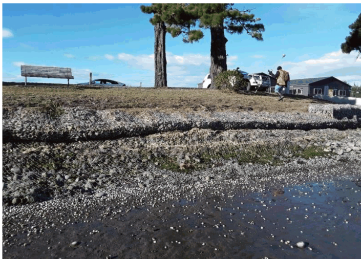
Figure 20: RM5-A upper layer of reno mattress added in 2017 to 10.8m elevation, with high ground up to 11.2m behind structure (Jacobs, 2019).
