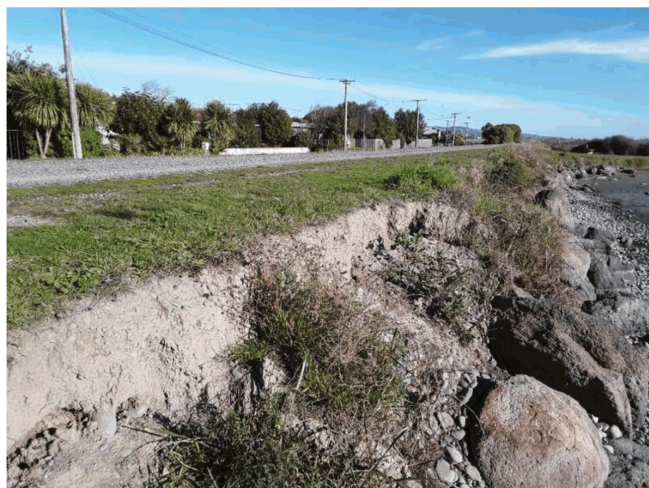
Figure 8: SB4-E Structure condition 'D' where front edge of the structure has shown significant erosion.
