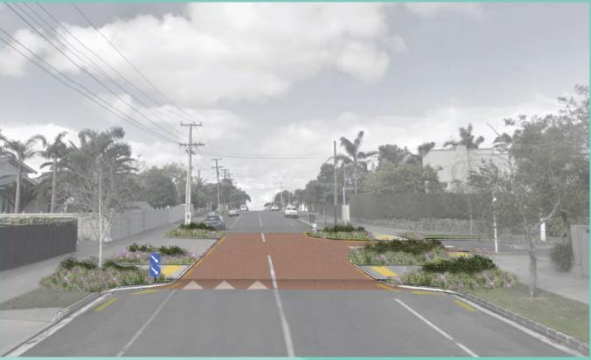
Raised intersection with improved pedestrian crossing facility
