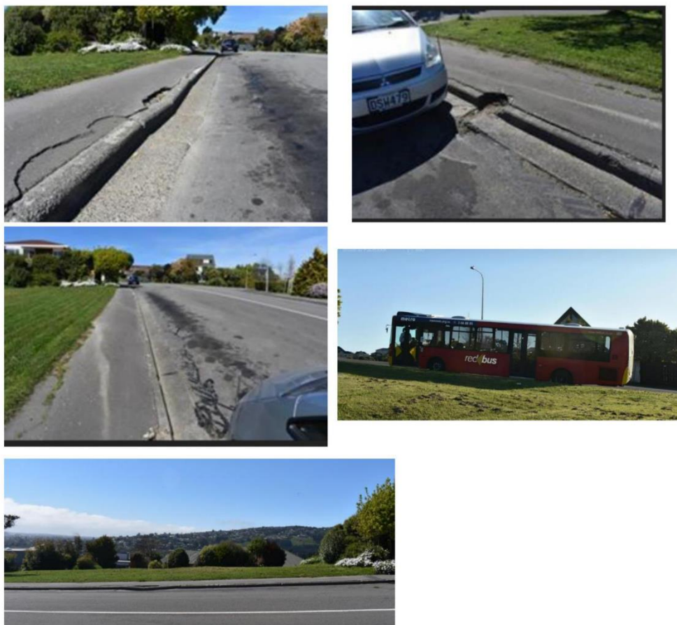
Figure 3: Photos of Damaged Kerb and Channel outside 63 Ravensdale Rise and Diesel Stains
