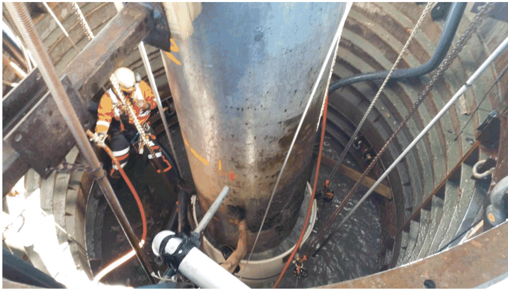
Figure 3: Inside the caisson – the top of the new steel jacket is visible in place around the column
