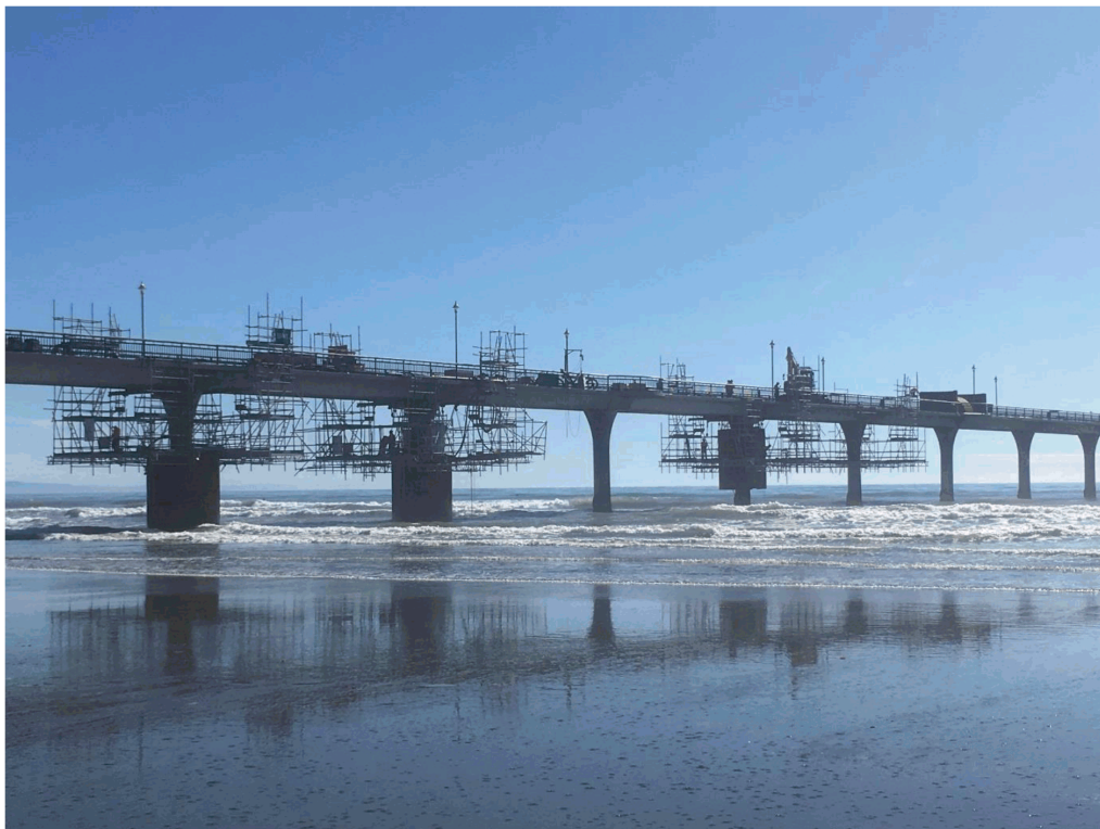
Figure 2: Temporary works - scaffolded access platforms, and caissons to access the damaged areas
