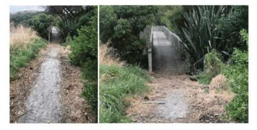
The last 5-10 m of the existing walkways will need to be lifted and the new link section added to sit about 500mm above the track. Overall about 70m of board walk will be needed to complete the exercise.
