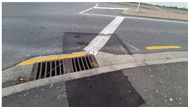
Figure 14 – Uneven Road Surface by the Double Sumps
