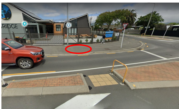
Figure 15 – Missing Warning and Directional Tactiles
