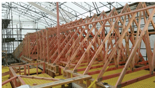
New Trusses being installed
