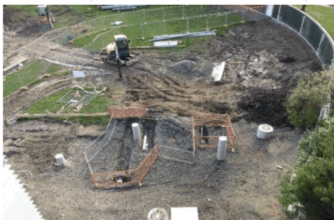
Indoor hydroslide foundations backfilled/balance tank piping
