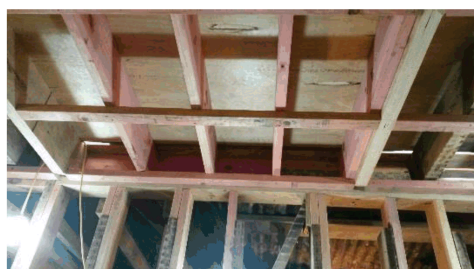
New replacement floor joists to the Ground Floor
