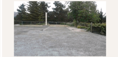
Godley House – Foundation Remediation- Heritage Banks Peninsula CB / December 2014
