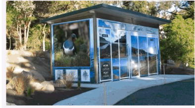
Pigeon Bay Campground Toilet - Banks Peninsula CB / 3 August 2016
