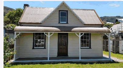
Grubb Cottage – EQ Repair and Maintenance- Heritage Banks Peninsula CB / 2 nd February 2016
