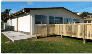
Duvuachelle Reserve and Campground - All Buildings Banks Peninsula CB / 30 th July 2015
