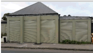
Akaroa Museum – EQ Repairs, Strengthening and Re-roof - Heritage Banks Peninsula CB / 13 October 2015
