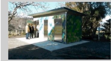
Duvuachelle Show Grounds Exeloo Toilet Banks Peninsula CB / 12 th August 2015
