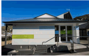
Lyttelton Mt Herbert Board Room Replacement (25 Canterbury Street) Banks Peninsula CB / 7 September 2016
