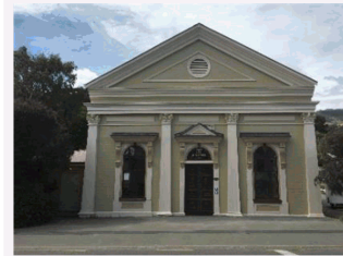
The Gaiety Hall – EQ Repair, Strengthening & Maintenance- Heritage Banks Peninsula CB / 1 st April 2016
