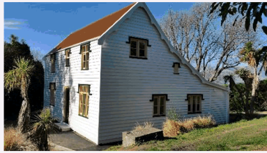
Governors Bay Headmasters House – EQ Repair, Strengthening and Maintenance- Heritage Banks Peninsula CB / 14 July 2016
