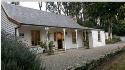
Stoddart Cottage – Earthquake repairs - Heritage Banks Peninsula CB / March 2017
