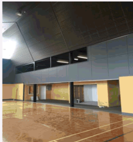
Lyttelton Recreation Centre and Trinity Hall Repair Banks Peninsula CB / Completed 18 th December 2015- Official Opening 20 th February 2016
