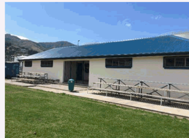
Lyttelton Recreation Ground – Pavilion and Shed #2 Banks Peninsula CB / 05 February 2016
