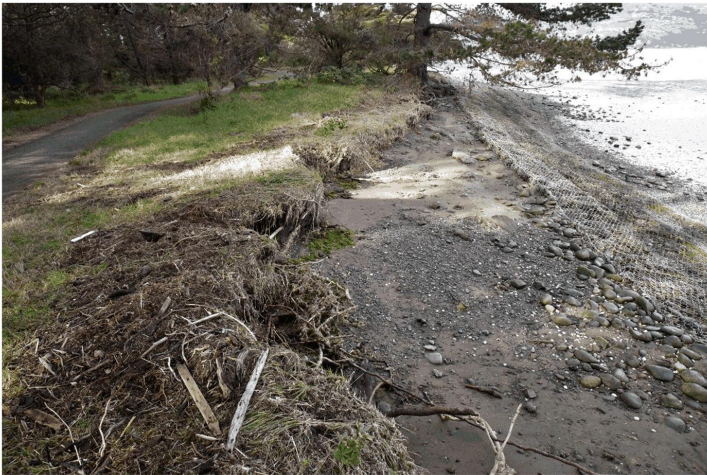
Figure 12 - Erosion in park behind existing reno mattresses
