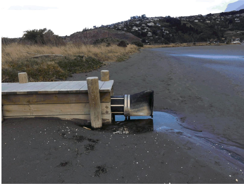
Figure 9 - Stormwater outlet with "duckbill" non-return valve in Southshore.
