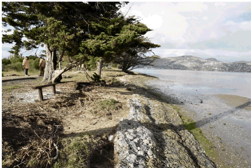
Figure 6 Beach Formation within South New Brighton Park behind Reno Mattress around Park Bench
