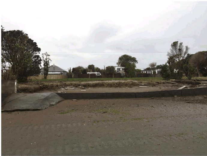
Figure 14 - Erosion behind old wall at Residential Red Zone on Rocking Horse Road
