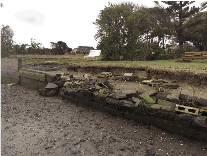
Figure 13 - Erosion behind rock armouring / old wall at Residential Red Zone on Rocking Horse Road
