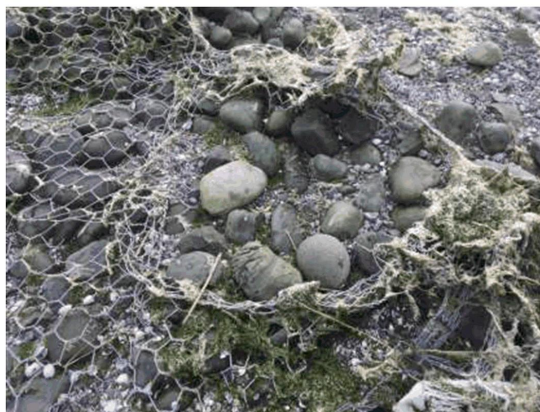
Figure 1 Damaged Reno-mattress
