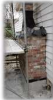
Reinstatement of Brick to Chimney
