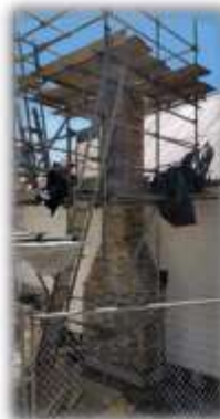
Brick Reinstatement nearing Completion
