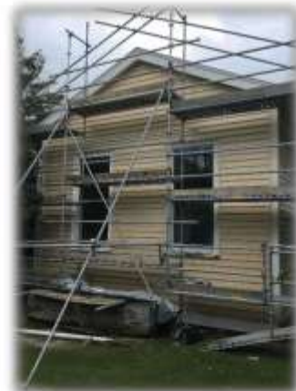
Replacement of weatherboards and painting has commenced
