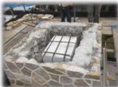
Tower capping strengthening
