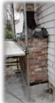
Reinstatement of Brick to Chimney
