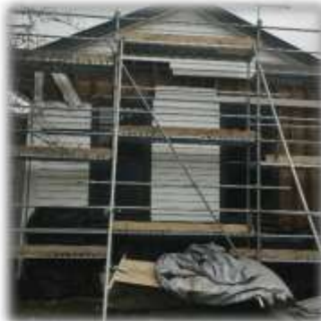
Replacement of weatherboards and painting has commenced
