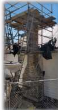
Brick Reinstatement nearing Completion
