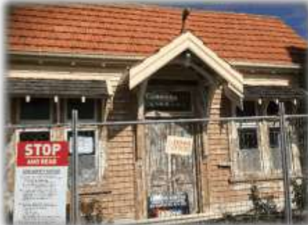
Exterior painting commenced with initial stripping
