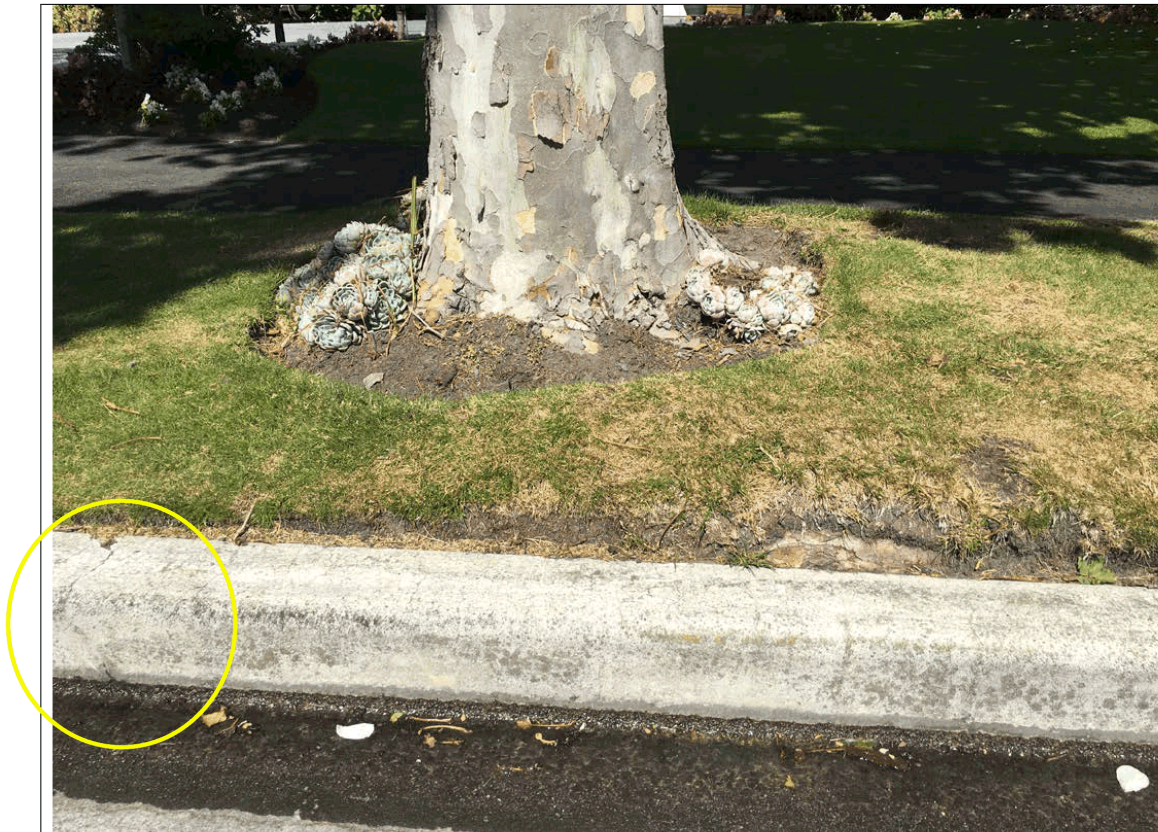
Figure 9: Showing location of (Tree 44826), in a narrow berm and the roots lifting the berm. Also cracking of kerb and channel immediately adjacent to the tree.
