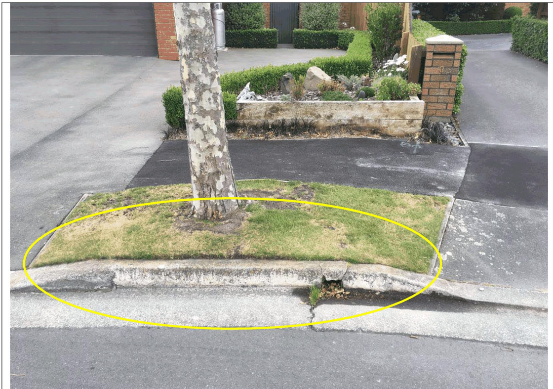
Figure 9: Showing location (Tree 44699), in a very small berm, the roots lifting the berm and cracking the kerbing above the stormwater outlet. Also in the background the recent footpath repair can be seen.
