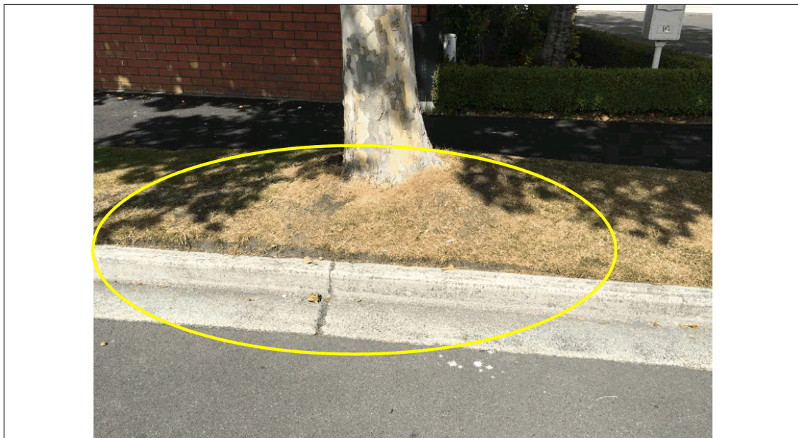
Figure 8: Showing base of trunk (Tree 44827) and roots lifting the berm adjacent to tree. Also cracking of kerb and channel immediately adjacent to the tree.
