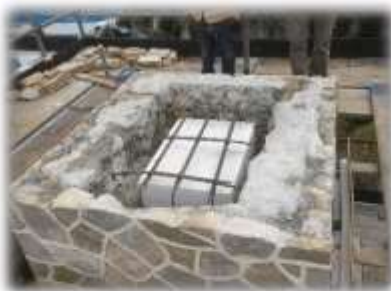
Tower capping strengthening
