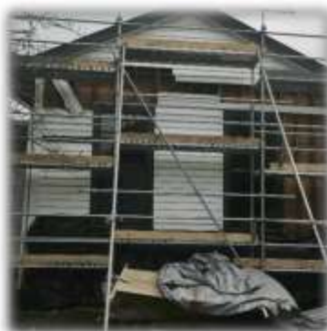
Replacement of weatherboards and painting has commenced
