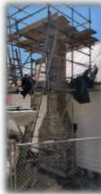
Brick Reinstatement nearing Completion
