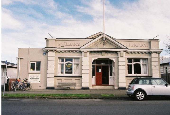
St Albans library pre-earthquakes
