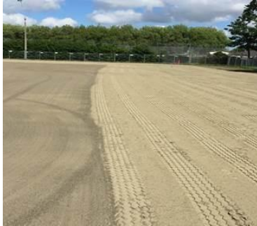
Turf Sand being spread, 22 November
