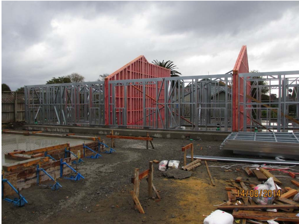
Figure 5: Knightsbridge Lane (8 x New Units) Foundations poured and framework under erection
