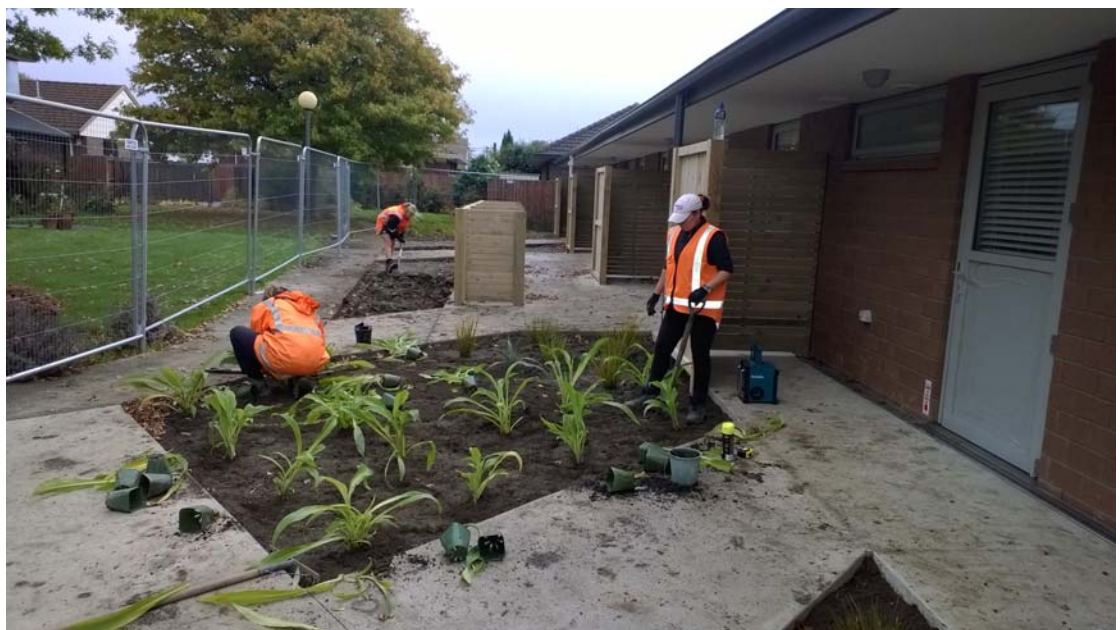
Figure 3: Dundee Place 12 x New Intensification Units Construction Progress (April 2014)
